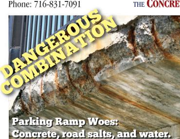
Designing, building, or maintaining a parking ramp in the Northeast can be a daunting task. Not only are there structural considerations, there is also the fact that in winter months vehicles constantly deposit water and road salts onto the surface. The water and road salts combined with the almost constant freeze thaw cycle that the ramp is exposed to can cause problems.
