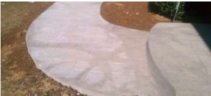
Discoloration due to curing covers that are placed on the concrete, some areas in contact with the concrete and others that are not. 4
