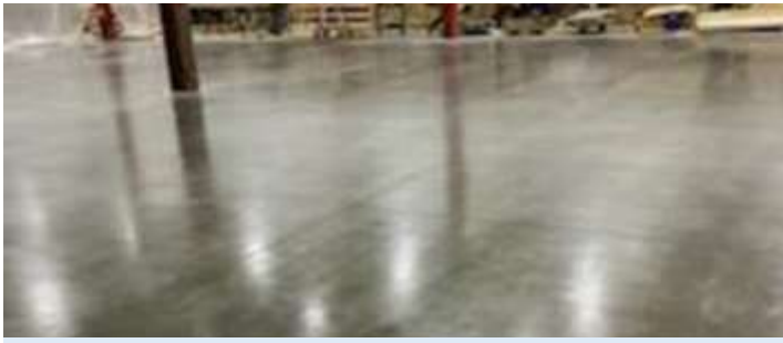
This concrete was overworked and thus the surface is darkened.
