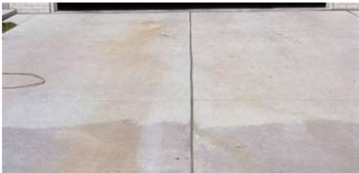
Discoloration of a slab with the darker area having the calcium chloride additive while the area closer to the door did not. 2
