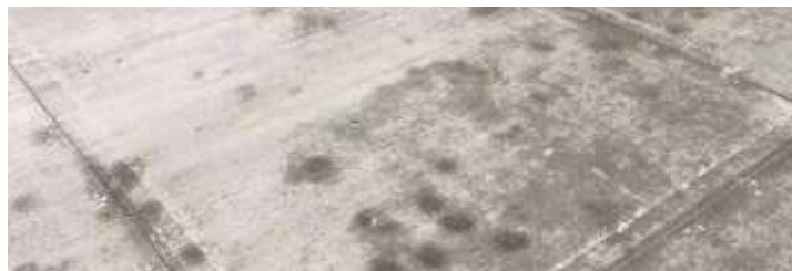
Example of blotchy and discolored concrete
