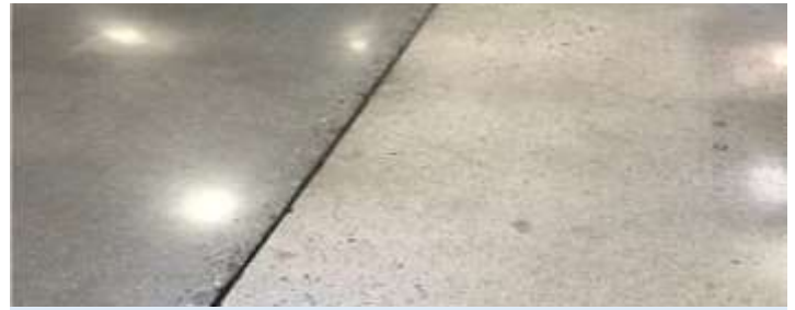
Two separate pours in the same room, possibly the result of the contractor getting concrete from two different plants/locations. 5
