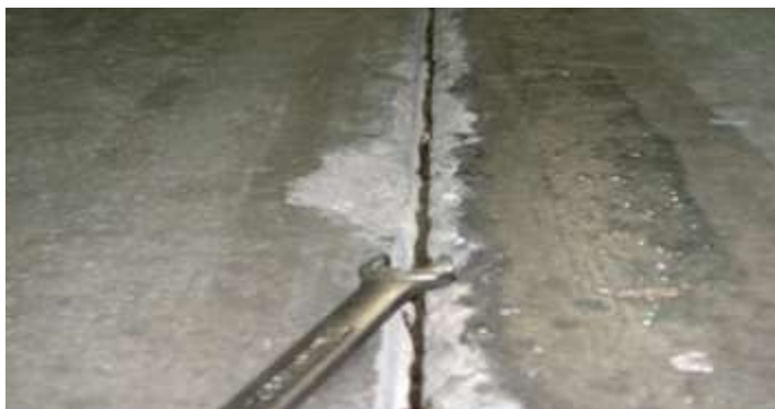
Control joint damage due to forklift traffic 4
