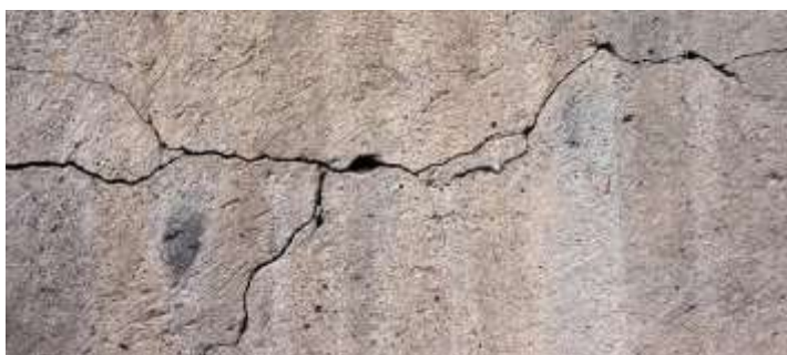
Random cracks in a concrete slab due to drying shrinkage 2
