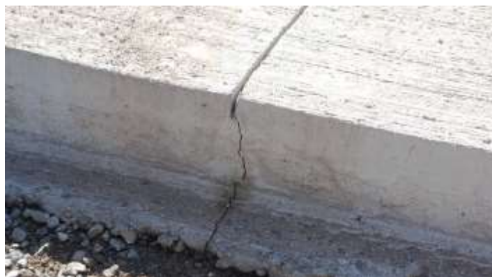
The cracking due to drying shrinkage happens along the weakened plane of the control joint cut in the slab 3
