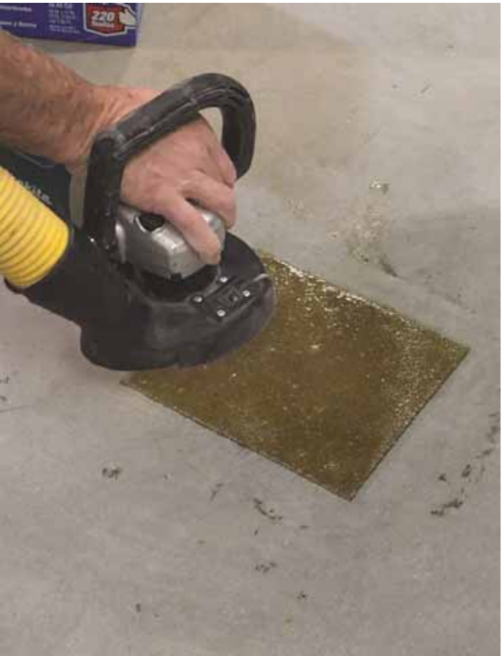
Grinding repaired area flush with the surrounding surface.
