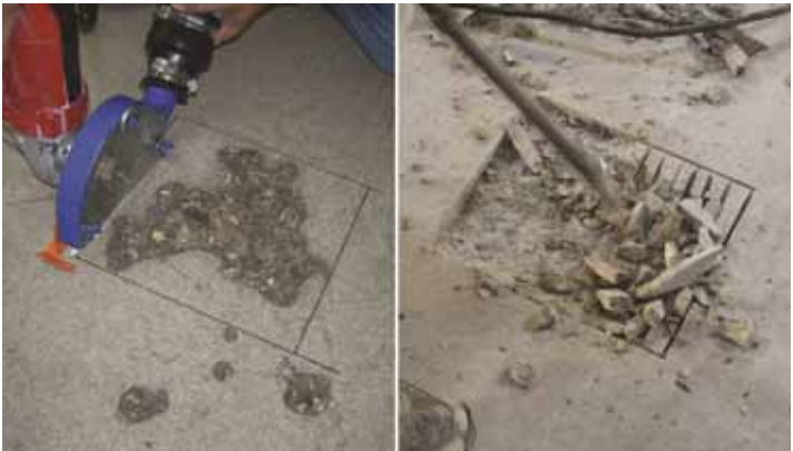
The preparation may be complex, requiring several steps to prepare the area for repair.
