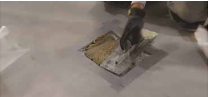
The material used in the repair is dictated by the size and depth of the damage and the floor use.
