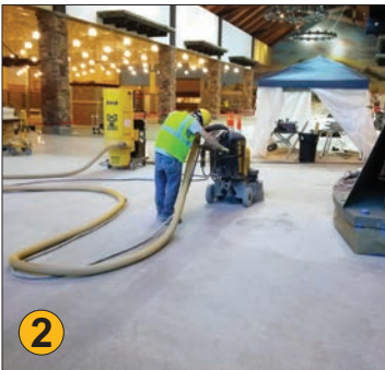
Photos: (1) (Top Right) Inside finished Cabela's store; (2) Initial grinding of new concrete, preparing for polish; (3) Section of polished concrete aisle; (4) Decorative concrete staining of intricate floor profile for waterfall exhibit; (5) Cabela's logo stenciled and stained by The MJA Company
