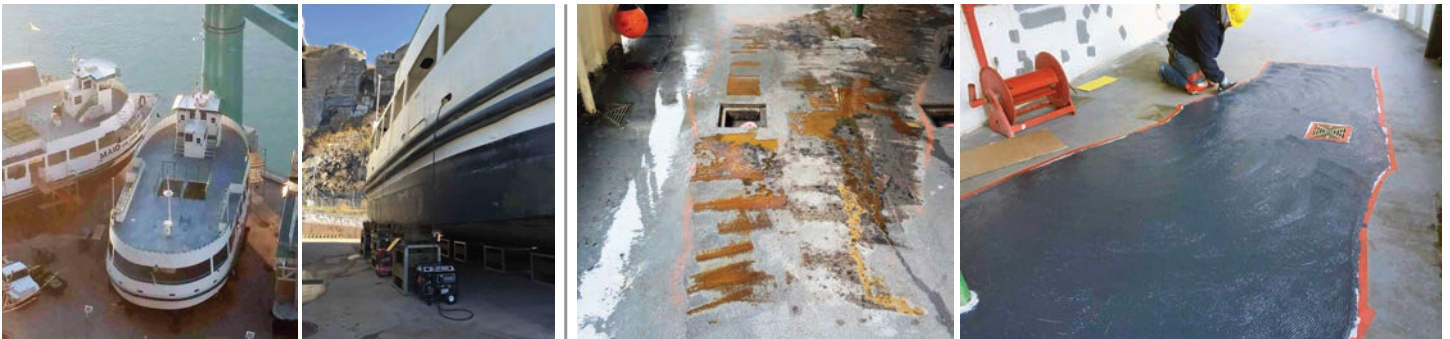
Maid of the Mist boats in dry-dock. Equipment and materials had to be hoisted into boats for project.
